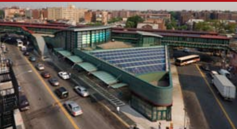
The Roosevelt Avenue Intermodal Station in Queens, New York is the busiest station in New York City's subway system outside of Manhattan, and features energy efficient systems, natural ventilation, conservation of materials and resources, and improved site management; transforming a utilitarian transit upgrade into a benchmark project for environmentally responsive design.
