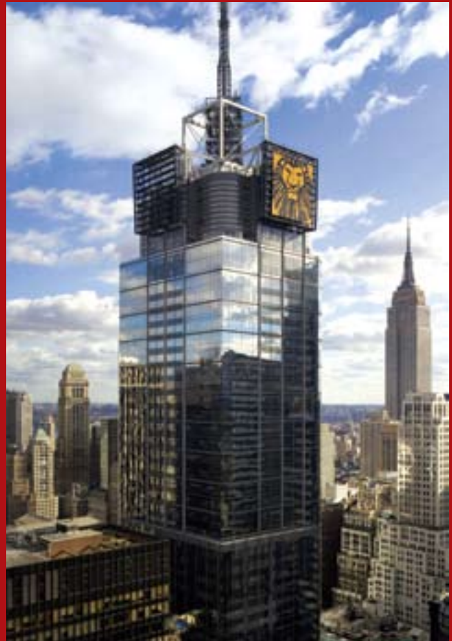
The 1,600,000 square foot Condé Nast Building at 4 Times Square is heralded as the first green skyscraper in the United States.
