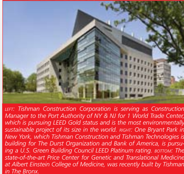
LEFT: Tishman Construction Corporation is serving as Construction Manager to the Port Authority of NY & NJ for 1 World Trade Center, which is pursuing LEED Gold status and is the most environmentally sustainable project of its size in the world. RIGHT: One Bryant Park in New York, which Tishman Construction and Tishman Technologies is building for The Durst Organization and Bank of America, is pursuing a U.S. Green Building Council LEED Platinum rating. ВОТТОМ: The state-of-the-art Price Center for Genetic and Translational Medicine at Albert Einstein College of Medicine, was recently built by Tishman in The Bronx.
